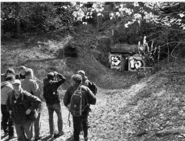
Main entrance to the Elephant. Two other doors are available; one is the emergency exit and the other is for ventilation. Photo Clive Penfold
